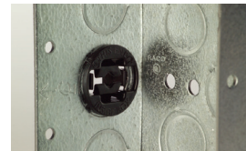
Step 2: Done - Ready for cable.
